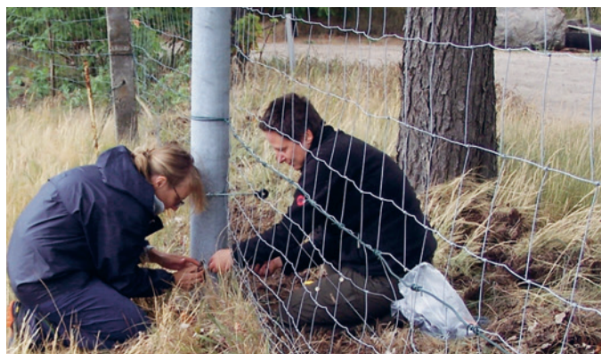
Fig. 1 Volunteers constructing protection to prevent predators getting under fencing. (Photo: S. Dittgen)
