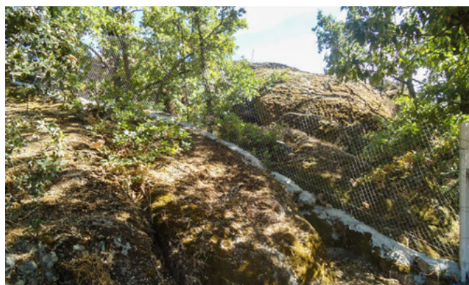
Fig. 7 Chain-link mesh fence at an ostrich farm with cement poles and concrete (masonry) base to prevent digging.
