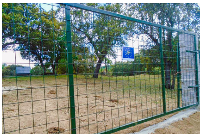
Fig. 6 Fencing to protect sheep and cattle from wolves, constructed from iron mesh welded panels, cement and granite poles and a concrete plinth under the gates to prevent digging.
